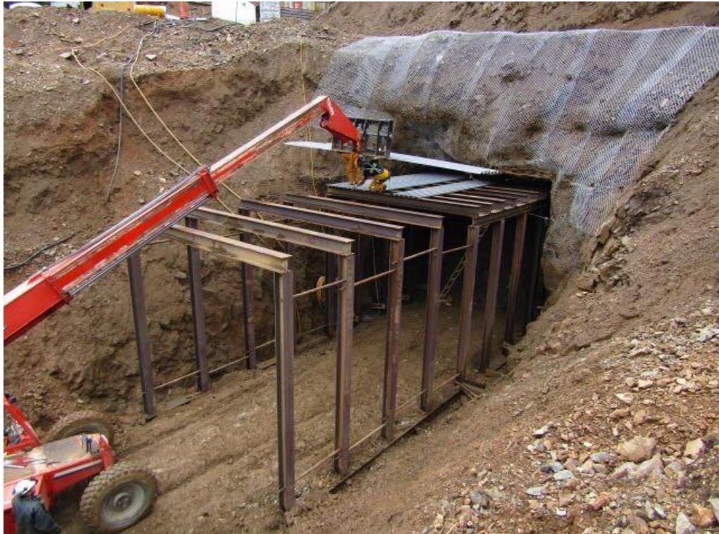
**Figure 3 : Installation of Bridge Sheeting on the Portal**
