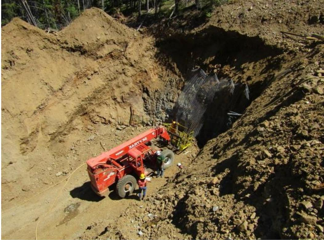
**Figure 1 : Excavation of the new Portal**
