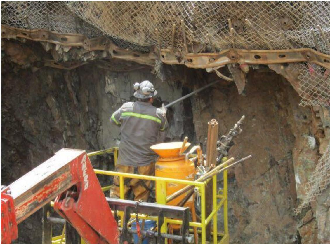
**Figure 2 : Scaling at the Portal**
