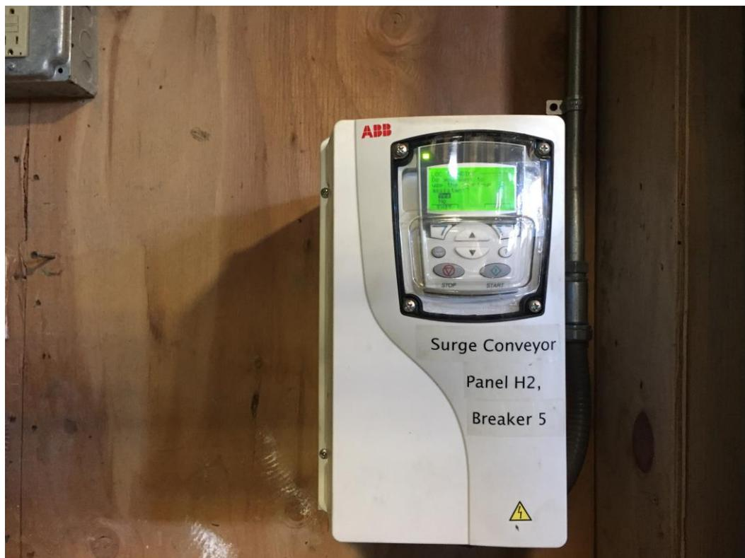
**Image 1: Belt feeder control unit. Communicates with Conveyor belt scale to ensure that only the desired tonnage is sent to the mill**
