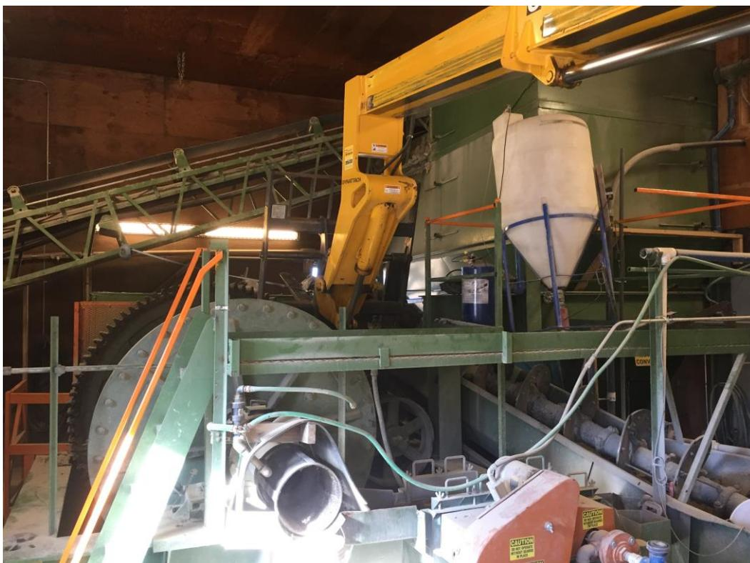
**Image 3: Telescope fork lift removing broken pinion gear from position**
