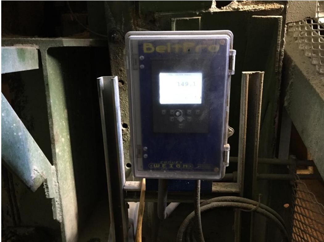
**Image 2: Conveyor belt scale determines the hourly tonnage required to be fed to the mill**
